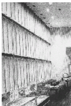
GA08. Rokkatei Makomanai Hall Vertical louvers serve as acoustic reflectors Hokkaido, Japan
