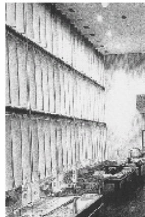
GA08. Rukkatei Makomanai Hall Vertical louvers serve as acoustic reflectors Hokkaido, Japan
